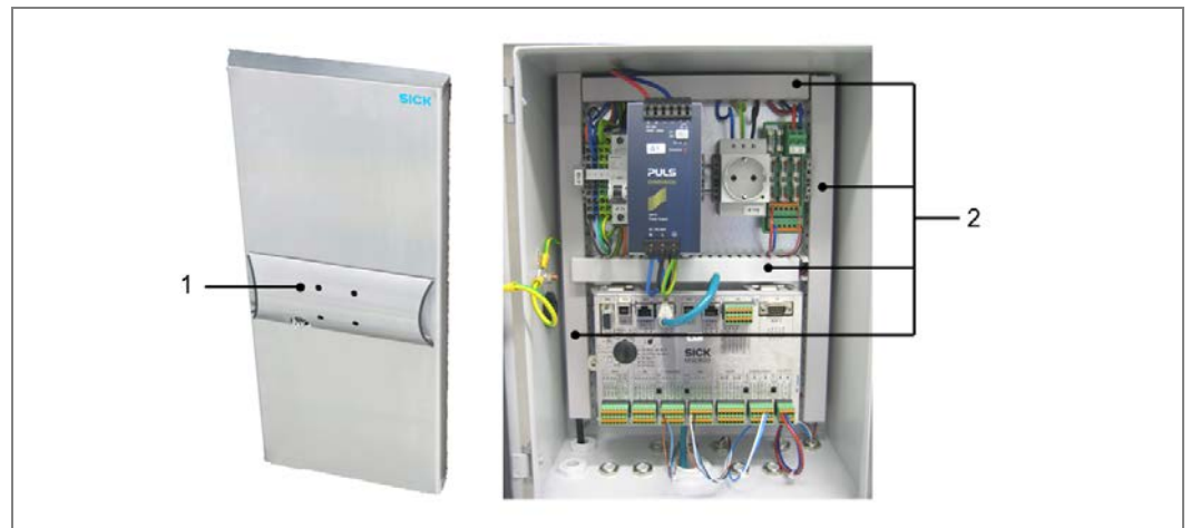
Fig. 35: Routing cables via cable channels
