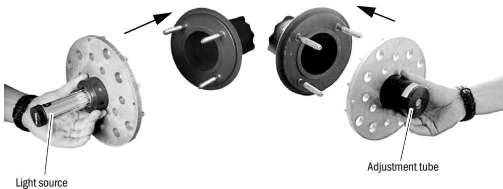
Fig. 5: Aligning the flange using an optical adjustment device
