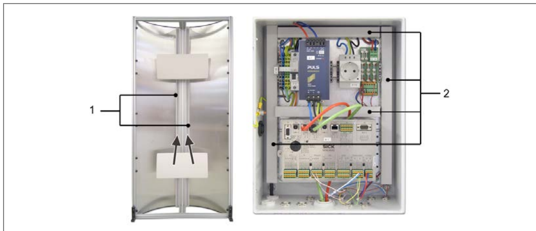
Fig. 34: Routing cables via cable channels
