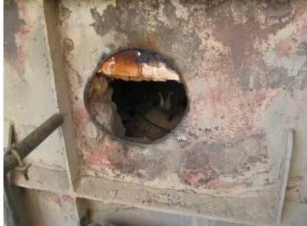
Fig. 20: Opening in the inlet chamber (example)
