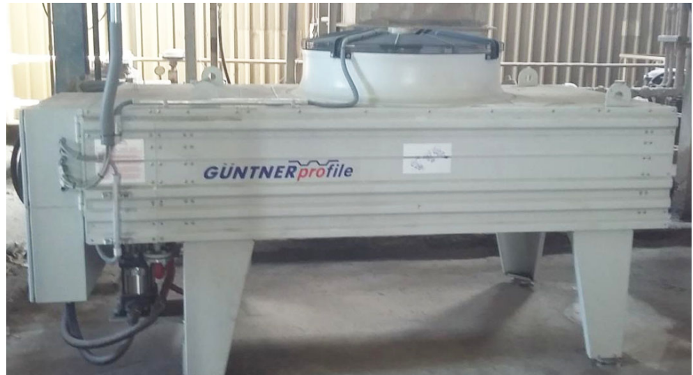
Fig. 40: Water to air cooling unit, completely installed
