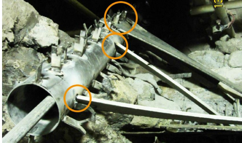
Fig. 23: Protection tube inside kiln secured with stabilizing material
