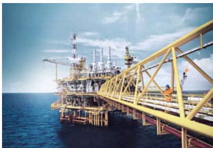
Flare gas measurement on offshore platforms ...
