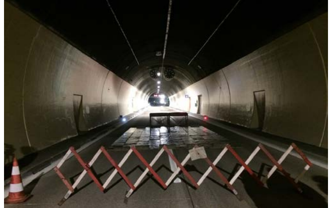
Image 4: Fire test location
