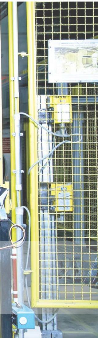
The deTec Ex II 3GD safety light curtains and the deTem Ex II 3GD multiple light beam safety devices from SICK meet the requirements of the ATEX guidelines for gas: II 3GD Ex nA op is IIB T4 GC X, and ATEX for dust: II 3GD Ex tc IIIB T135°C Dc. Both products provide maximum reliability and a very high level of safety for employees – even in explosive environments.
