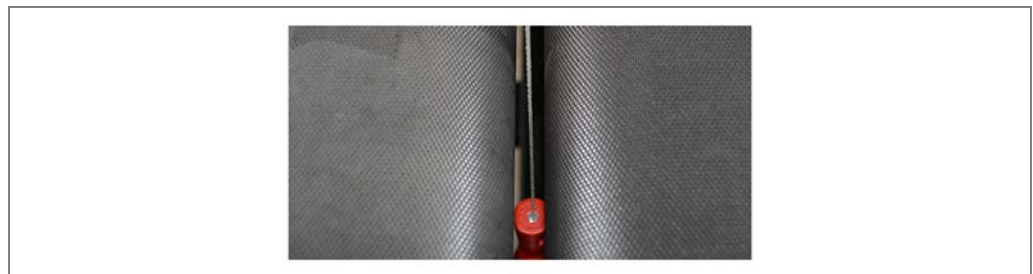
Fig. 53: Plumbline in the center of the gap
