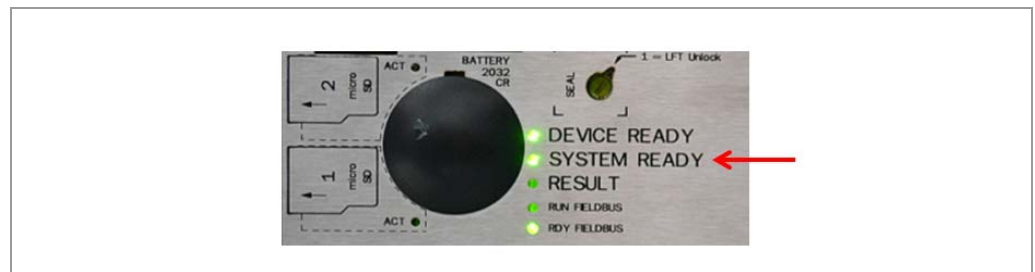
Fig. 146: MSC800 fault situation: “SYSTEM READY” LED does not light up
