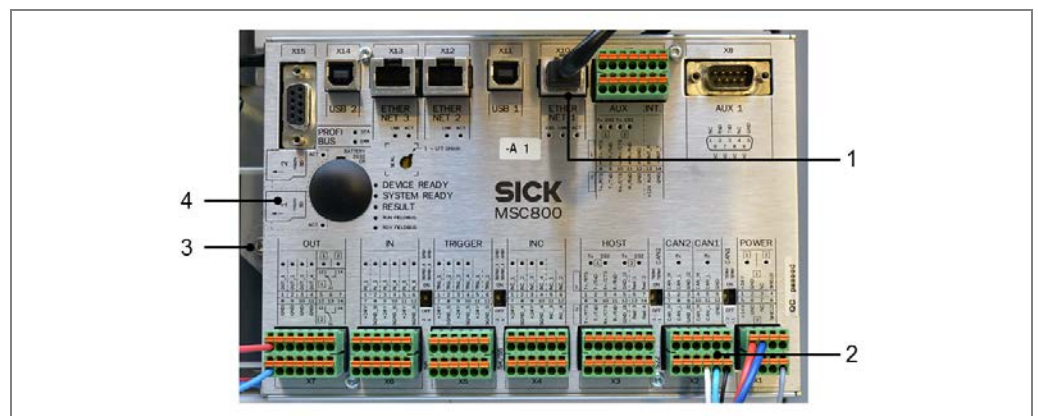
Fig. 92: Unplugging the cables and terminal blocks from the controller
